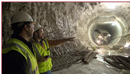
Trades workers involved in a Chicago Water Reclamation District sewer project.
