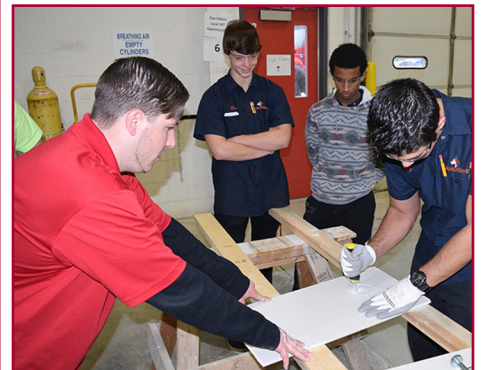
Carpenters Assistant Apprenticeship Coordinator Nick Sanfilippo helps a student cut a circular hole through wall board before it is fastened to a frame.
