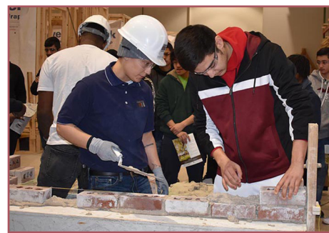
Bricklayers Pre-job apprentice Julia De La Cruz shows a student how to keep the bricks on the plumb line.
