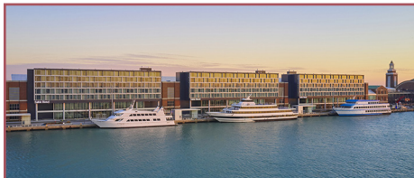
New Construction Chicago winner in 2020 - Navy Pier Hotel & Rooftop Venue.
